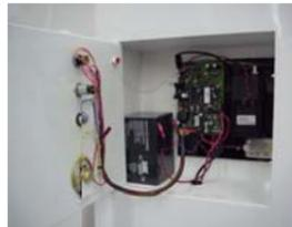
Next, check that the microphone and harness cables are still connected to the faceplate as shown below
